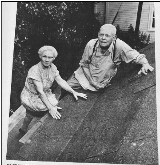
IN HIGH PLACES: Mr. and Mrs. William H. Kimball of Grove Street are re-shingling their three-stall garage—all of 40 feet high with a 60-degree pitched roof. Mrs. Kimball is 71 and her husband is 90 years old. Activity is one of Mrs. Kimball's recipes for longevity. (Photo by Shu)
